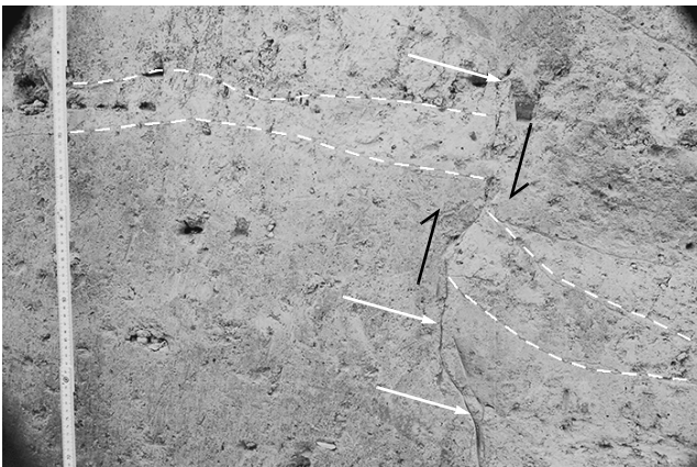
Fig. 17. Sagging of the central fragment of wall at f.s. 5 (Fig. 10) along the extended fracture is documented by displacement of the yellow loess-like loam bed. The direction of displacement is shown by black arrows.
